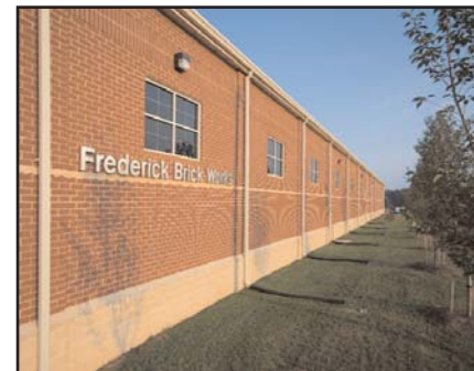
Frederick Brick Works' masonry veneer
