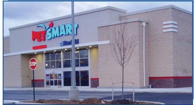
Chambersburg Crossing, Chambersburg, PA
